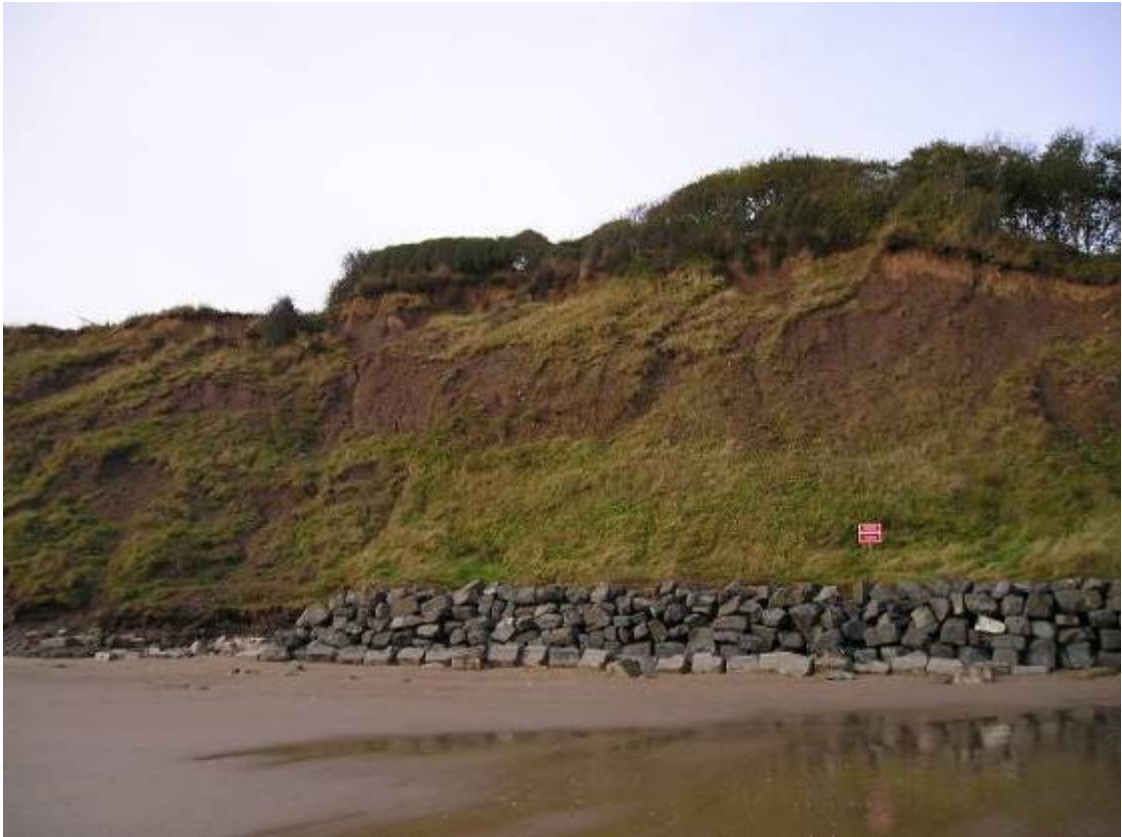
Figure 32 – Cliff Erosion in Filey Bay (Marker 5 is located to the left, beyond the extent of the rock armour)
